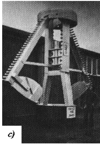
Figure 1-3 a) hydraulic rotary drilling equipment b) C.F.A, c) underreaming tool open position
